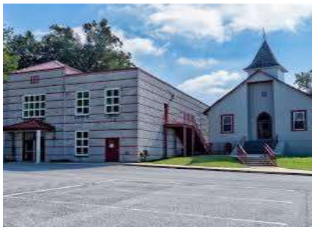
St. Stephen AME Church (Outside of CT)
