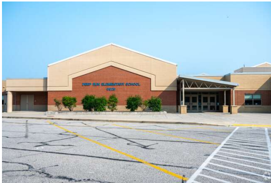
Deep Run Elementary School and School-Based Wellness Center
